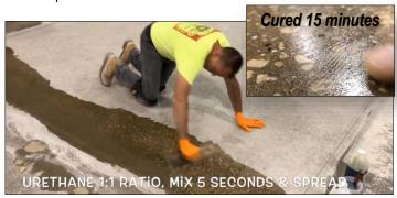
Deep voids should be filled with dry sand to bulk up the depression and reduce product from leaking through cavities. Should any sink holes occur, reapply Smith's Poly PCF-45 as necessary once the crack filler has hardened for approximately 10 to 20 minutes to allow the first layer to begin to gel and begin to seal off the holes causing the leak.
