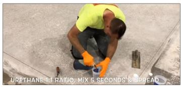
APPLICATION: Once mixed, work quickly to pour out the mixed Smith's Poly PCF-45 slightly overfilling the voids with the intent to diamond grind smooth when hard cured. A finishing trowel or drywall tape knife may be used for patching and skim-coating applications. Dependent upon the depth of cracks, holes and voids, may be filled in 1 or 2 pours with 10 to 20 minutes between lifts.
